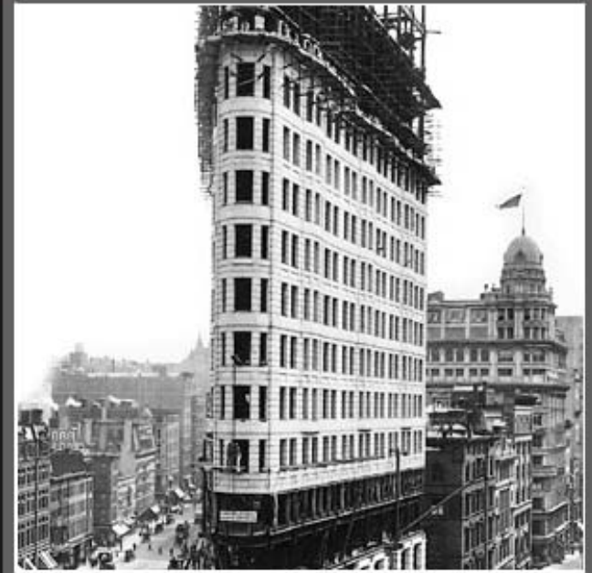
🔍 Flatiron building under construction in New York City (finished in 1902).
